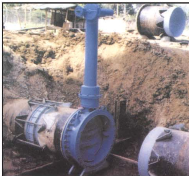
Gunric Valve being Installed in Thailand
